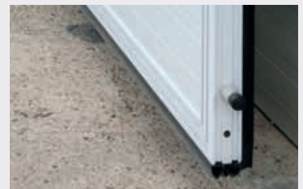
Detail of side and bottom sealing joints.
