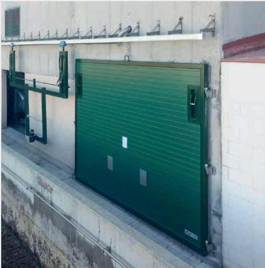
Detail of side and bottom sealing joints.
